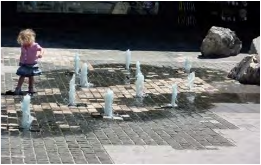
Cobble feature paving and in-ground water feature
