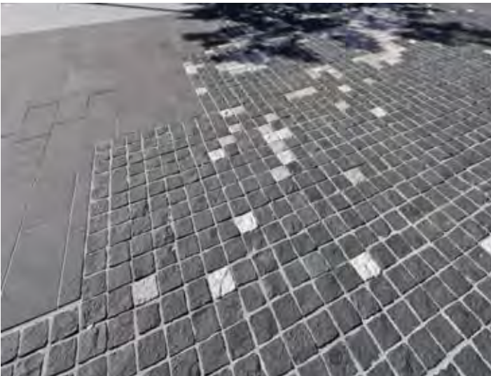
Cobble feature paving
