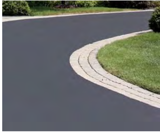
Hot mix asphalt pavement
