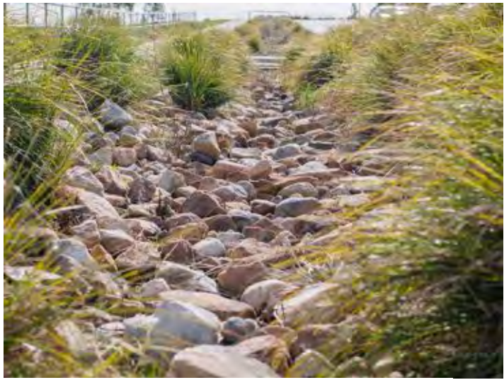
Rocky areas within bioretention basin
