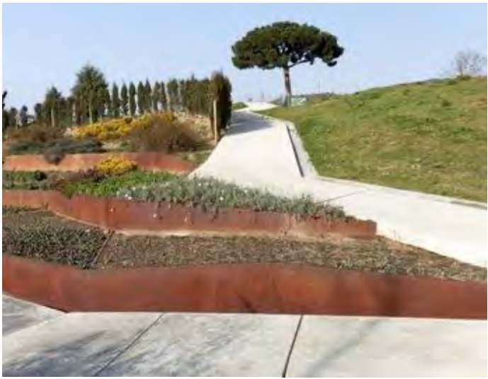
Corten garden retaining
